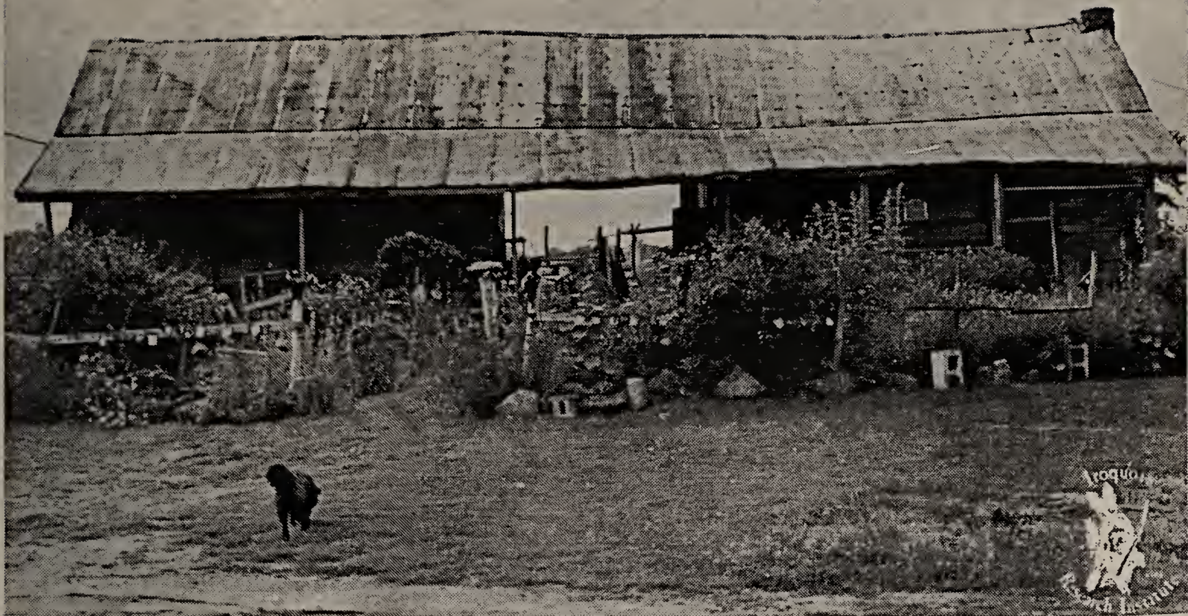
Plate 7. The dogtrot. The dogtrot house type, illustrated above by a mid-nineteenth century example near Earle, Arkansas, is almost always of log construction. The natural taper of a log and its tendency to fail by shearing forces indicated that log construction was inappropriate for even moderately large buildings. The dogtrot represents a successful attempt to overcome the limitations of a building material.
